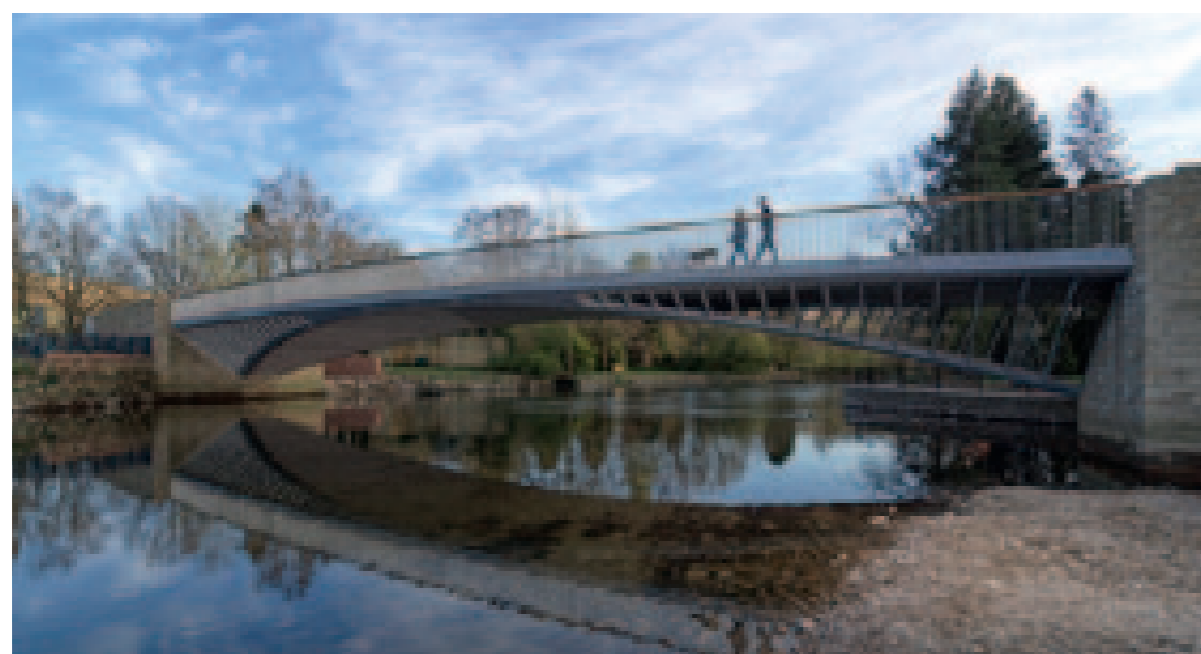
Example of new bridge constructed within historic setting at Pooley Bridge, Penrith (©Sean Coby)
